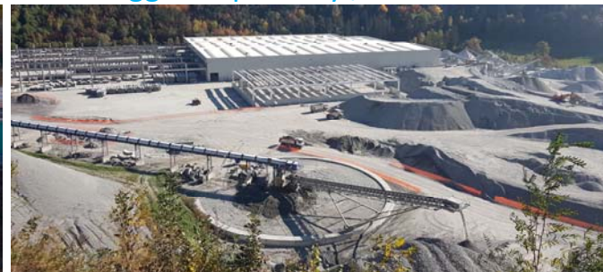
Hinterrigger repository / construction site
