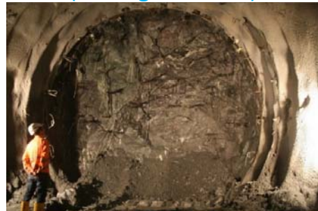
Exploratory tunnel (Mining methods)
