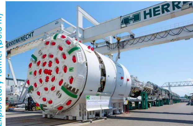
Exploratory Tunnel (Ø6.8 m)
