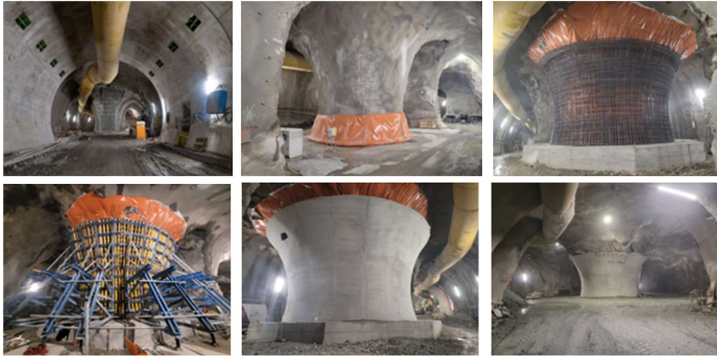
Figure 13. Underground roundabout construction phases: upper left- phase 2; upper center - phase 3; upper right, bottom left and bottom center - phase 4; bottom right - phases 5-7 (property of the authors).
