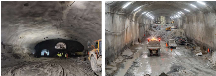
Figure 14. Car parking cavern ongoing excavation phases (property of the authors).
