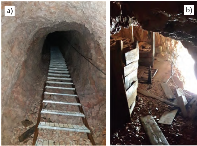
Figure 15. (a) Castelletto tunnel. (b) Access to Castelletto tunnel (authors' photos).
