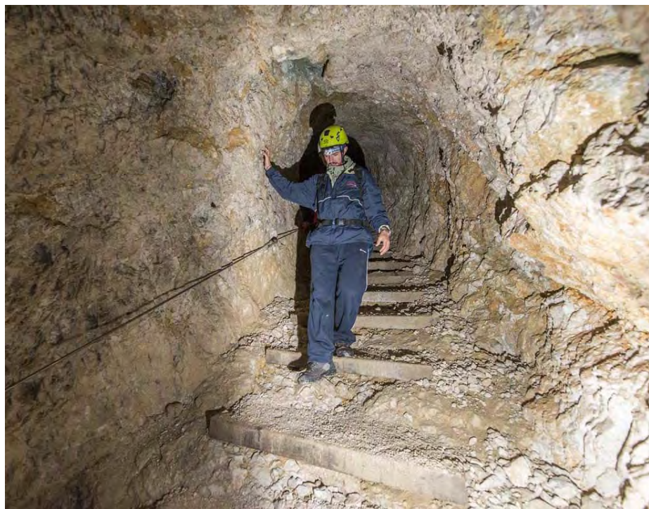
LAGAZUOI TUNNEL (PHOTO BY GIACOMO POMPANIN)
